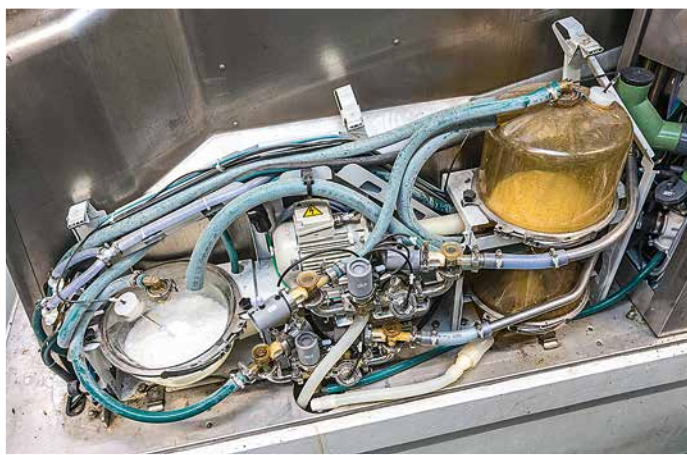
Each GEA robot has a reservoir for the milk destined for the bulk tank and a reservoir for separated milk. This reduces the number of necessary cleanings when cows are undergoing treatment.
